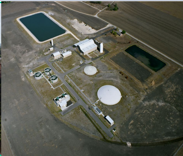
East Williamson County Water System
